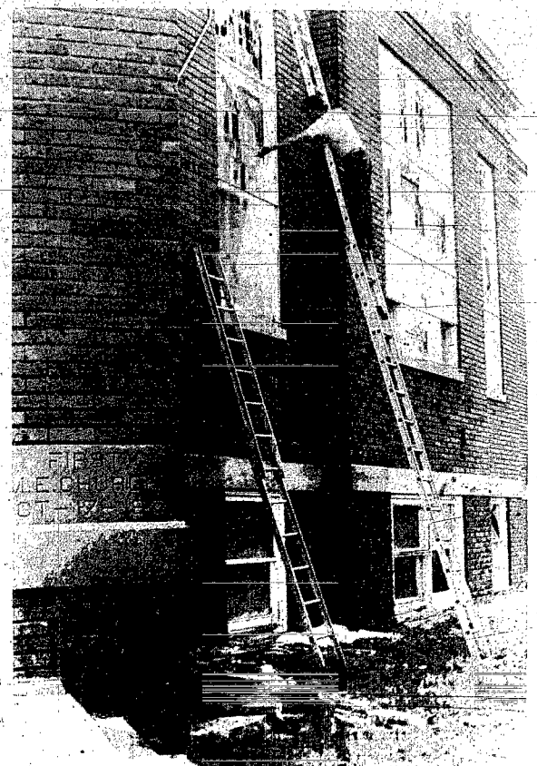
PICKING UP THE pieces of stained glass from the Methodist church in Allen, S.W. Moynihan. The windows were shattered in a hail storm that hit the area Saturday morning. It permeated the premises and smashed the stained glass windows.
